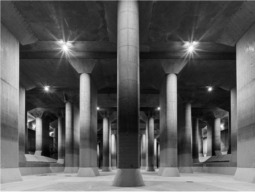
FIGURE 15.1. Water Chamber. Inside the 248,508 cubic feet water chamber, are five-dozen 60-foot high pillars, each reinforced by five hundred tons of concrete. Released under the GNU Free Documentation License.
