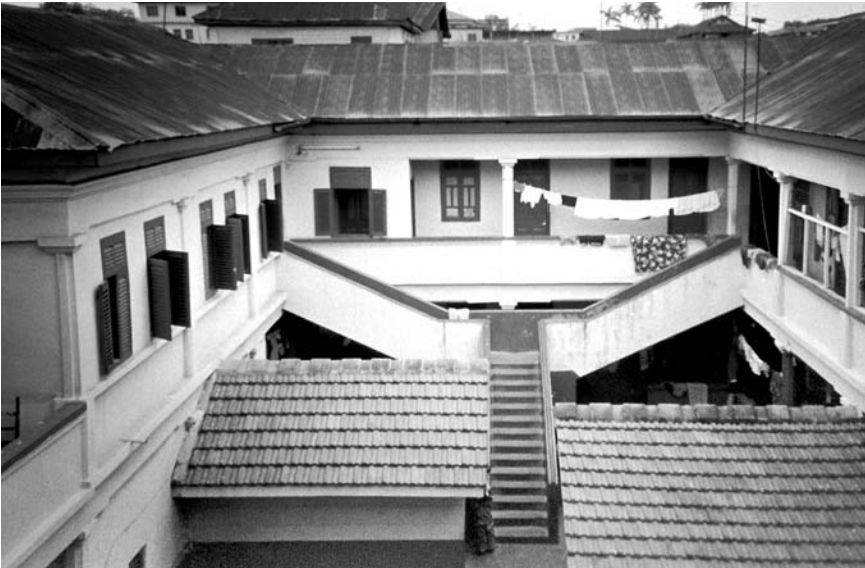
Family house of President Kufuor in Kumasi, Ghana. This house is less than five hundred metres from the Asante king's Manhyia Palace (photo by D. Ray).
