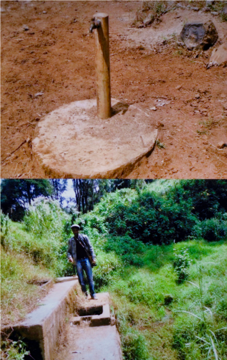
FIGURE 7.2. Dilapidated Water Catchment Tank and Abandoned Stand Tap Due to Poor Management in Ngarum-Ndu Municipality, Rural North-West Cameroon. Photo by Henry Bikiwibili Tantoh.
