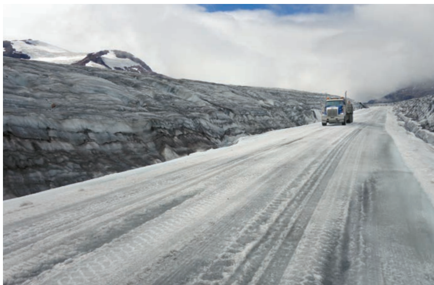
Figure 2: Glacier road over the Knipple Glacier in northwest British Columbia that leads to the Brucejack Mine. Photo: A. Bevington
